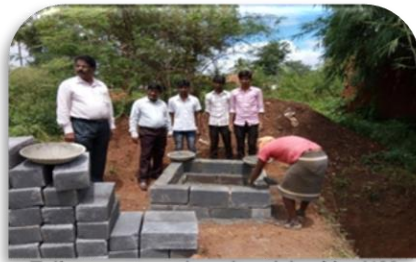
Toilet construction site visited by NSS Program Co-ordinator Dr. M. B. Dalapati.
